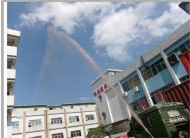
Fire hydrant test
